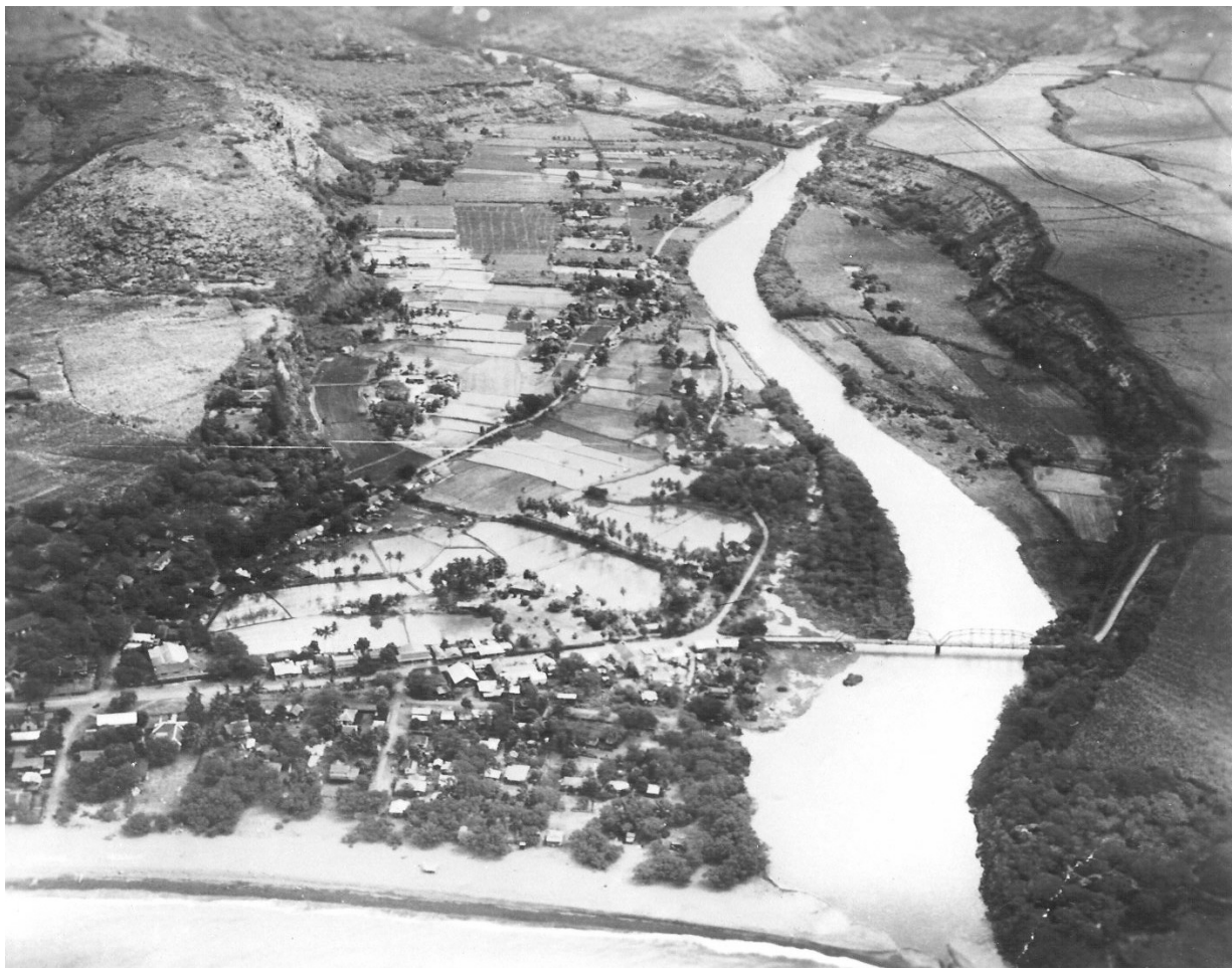
Photo: View of Waimea Valley, 1926. At the top photograph can be seen the branching of the river. To the right is Makaweli River and to the left is Waimea River and to the left of the branching of the river is the ridge that Menehune Ditch wraps around. The result is fertile fields below. The bridge and Waimea Town itself are located in the lower section. The road into town is Waimea Road. The Russian fort is at the river mouth to the right under the trees.
